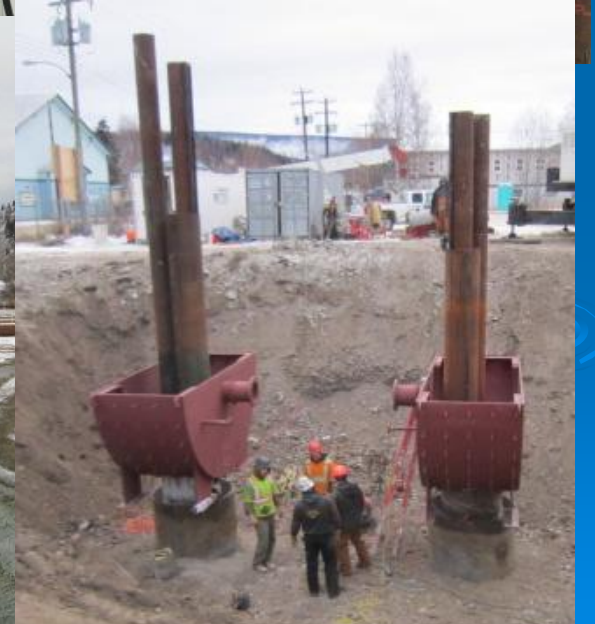
Two bioreactors extending 100 metres into the ground
